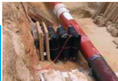
Lifting and leveling of pipelines - Construction -
