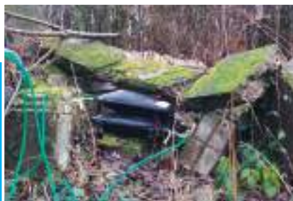
Lifting of blocks Stone, extrication - Civil Protection -
